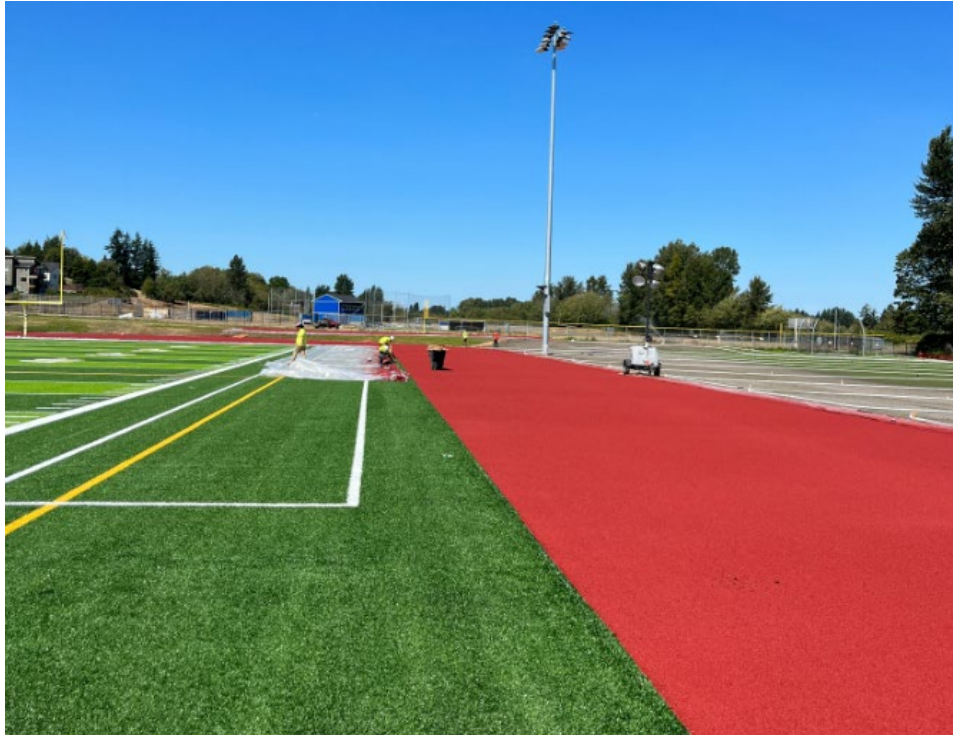
Rubberized track surface installation. Striping to come.
